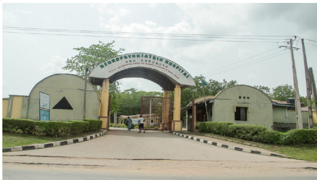
Figure 1: Picture of the New Psychiatric Hospital, Aro, Abeokuta.
